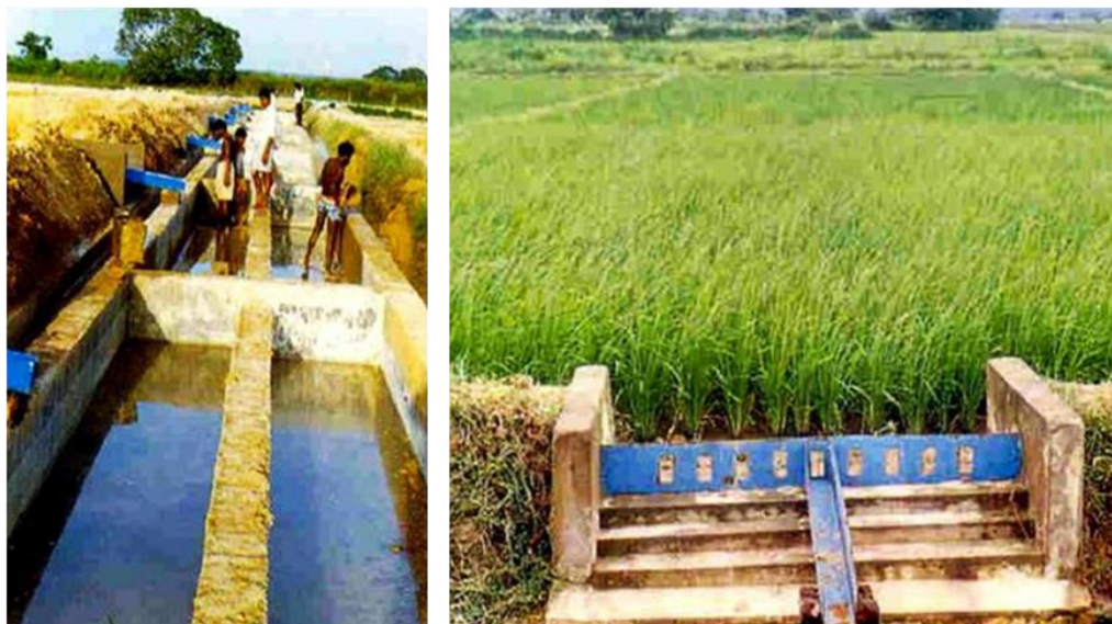
Figure 5.3. Increased dyke height for in-situ rainwater conservation. Source: http://www.iiwm.res.in/technology.php
